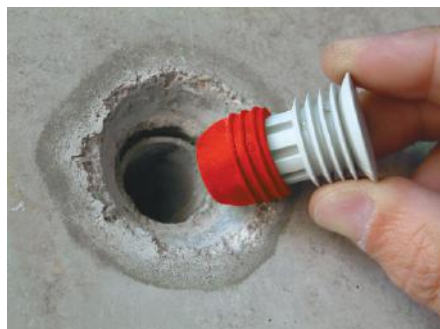
1. Insert the Solco Form-Tie Plug into the open end of the conduit sleeve.
