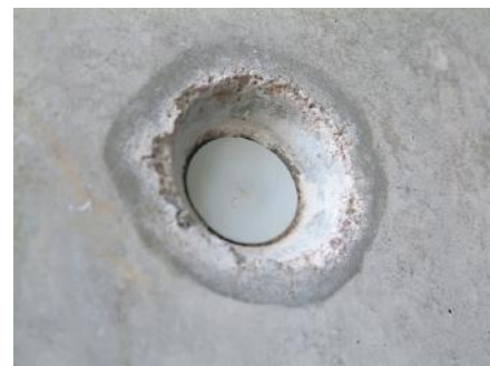
3. The Solco Form-Tie Plug installed. No further finishing is required.
